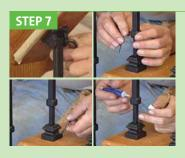
Once the baluster is installed, tighten and lock the baluster base, telescopic shaft and swivel top with the set screw. It is suggested to apply thread locking liquid on the set screws. Do not apply thread lock liquid on the swivel top until it is securely screwed into the handrail.
